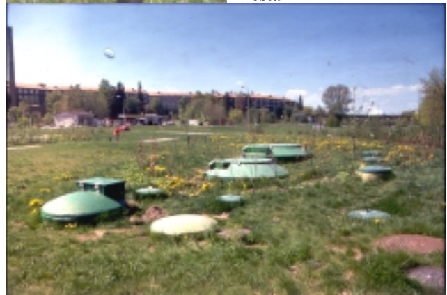
Fig. 38 - Only the tops of the tanks show in Understenshojden's system
