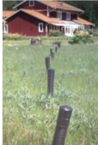
Fig. 37 - All that is visible of the soil infiltration bed in Akesta
