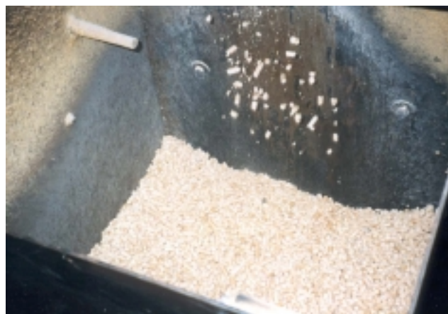
Fig. 24 - Hopper for wood pellets at Tuggelite
