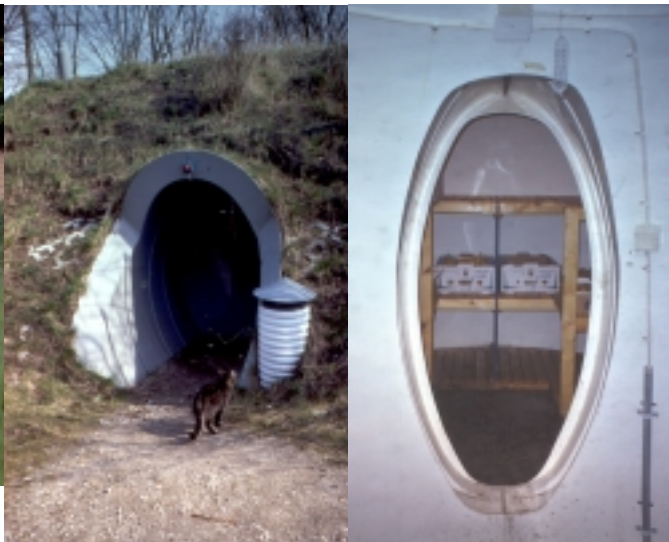
Fig. 11 - South facing fiberglass root cellar in Solbyn tends to overheat
