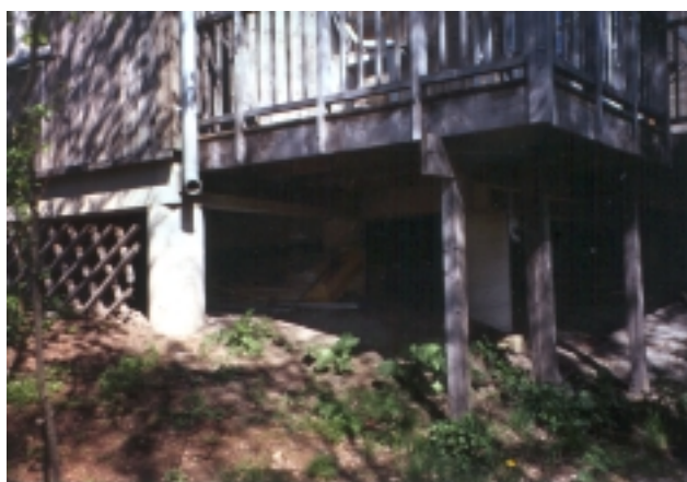
Fig. 19 - Homes in Understenshöjden are on stilts in order to minimize the impact on the site
