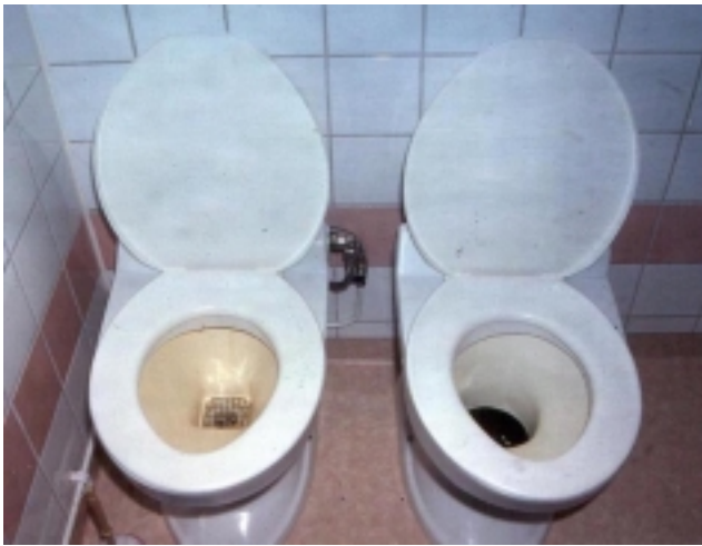
Fig. 31 - Toilets adapted for urine and compost
