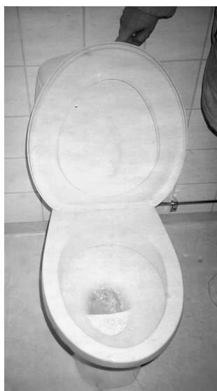
Fig. 33 - Urine collection inadequate
